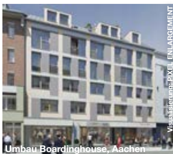
Umbau Boardinghouse, Aachen
